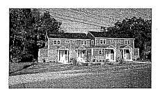
Two model buildings were renovated in 2016. The renovation allowed for the inclusion of energy improvements and greater amenities within the units. The buildings were completely renovated to meet Energy-Star Standards. Improvements included replacement to high efficiency windows throughout, new doors and insulation. Interior construction included the addition of a half bath and laundry on the first floor, new kitchen cabinets and countertops, new
